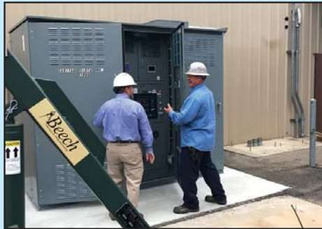
Maintenance work at the Pump plant.
